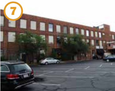
7 Dilworth Artisan Station Camden Square Rows of windows on the building
