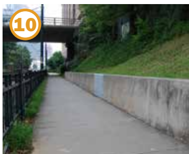
10 Carson Station City Loop Retaining wall leading up to Morehead bridge
