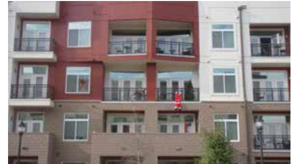
South End Apartment Balconies
